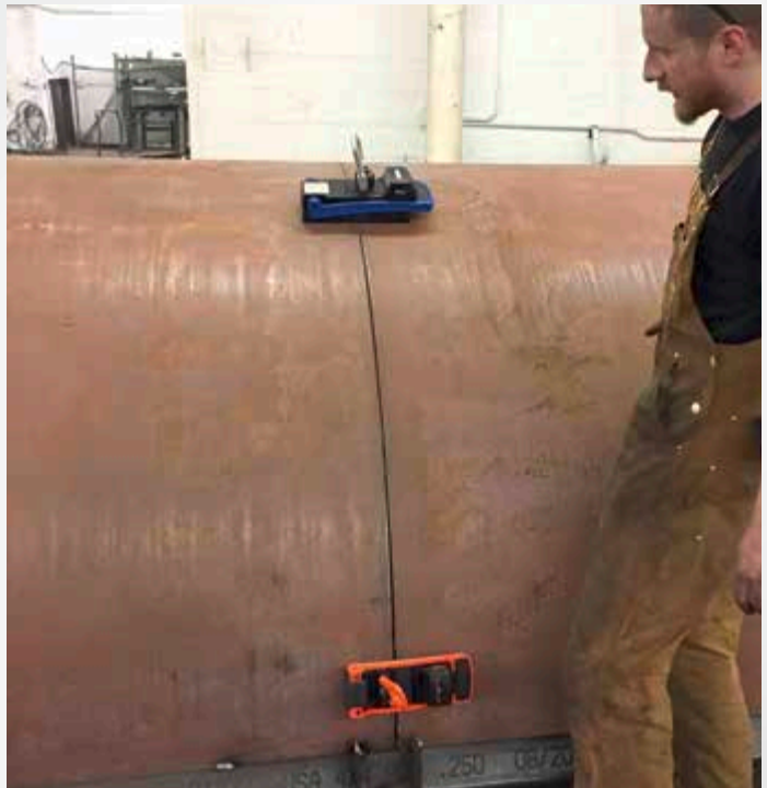
CONTAINER CONSTRUCTION–WROCLAW/POLAND – MAREK
