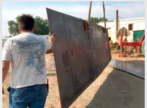
HALL CONSTRUCTION- BLOOMFIELD/USA – RICARDO
